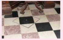
Three pipes conduct sound through the floor into the King's winter room. Pipes are covered when not in use.
